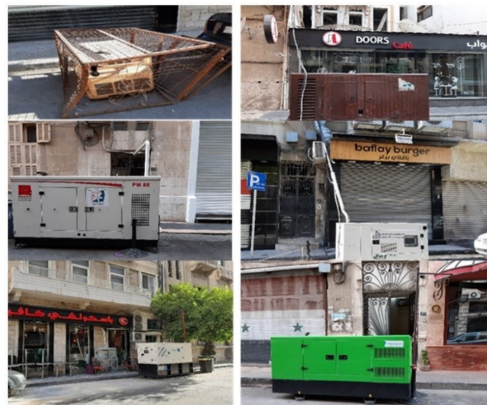
Fig. 4: Six diesel generators used by restaurants and shops located along the street. These generators operate during the periods, when there is no electricity.
